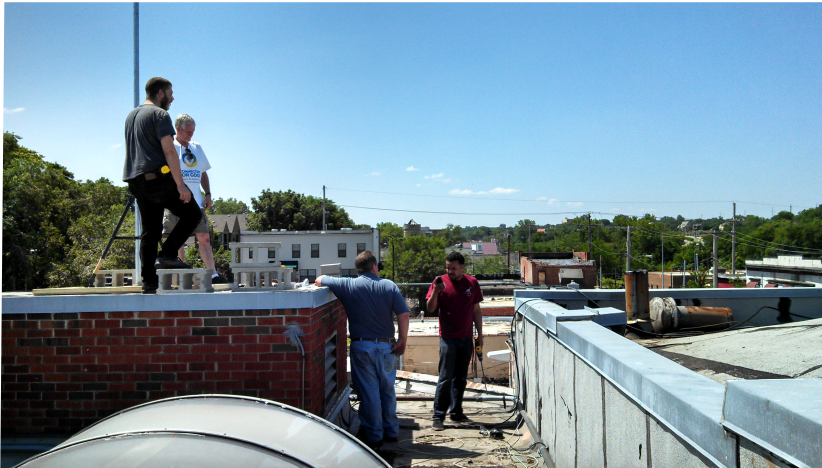
Isaac and Clint installing KCFN gear with Dan Harmon and Rick Deane of Connecting for Good.
