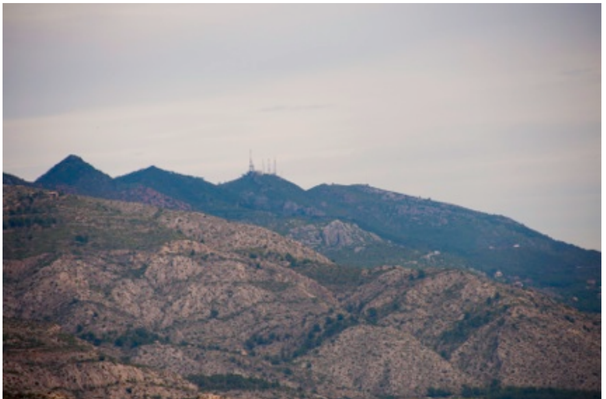
A telephoto picture of the radio towers on the distant ridge
